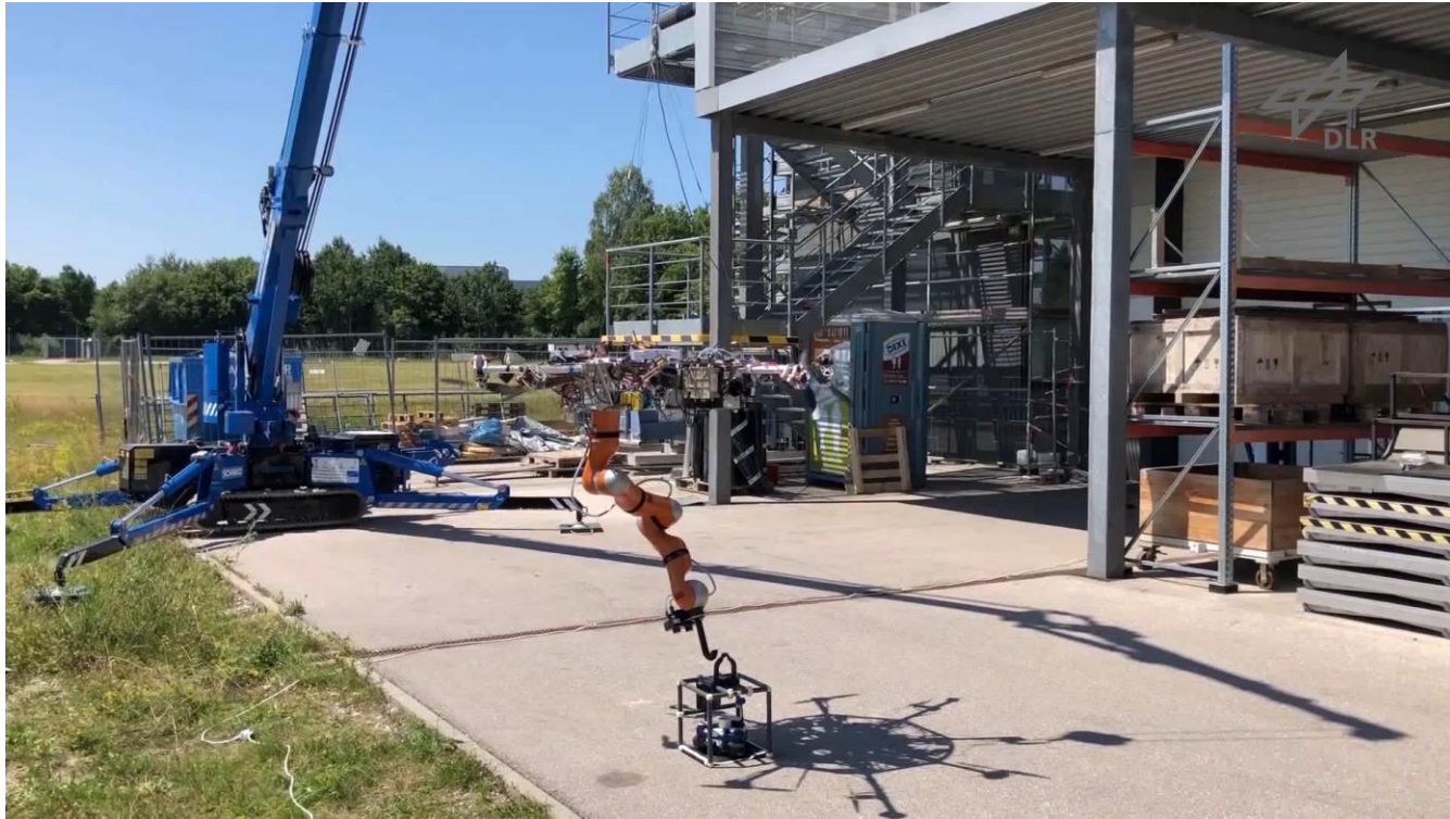
Deployment and Retrieval of Inspection Robotic Crawler [1]
